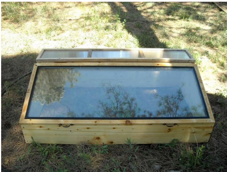
Figure 39: Structure #2 – Cold Frame with Foam Board Insulated Walls
